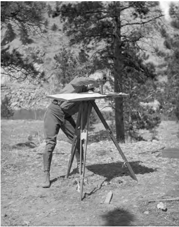
Figure 1—Arthur Carhart at his plane table, Trappers Lake, 1919. The photograph is used with the permission of The Library of Western History, Denver Public Library.
