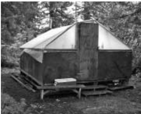
Figure 4—Moose hunters can apply for special use permits to construct tent platforms for use during the season, but must then collapse the structure and may store materials on site year-round. Photo by John Hendee.
